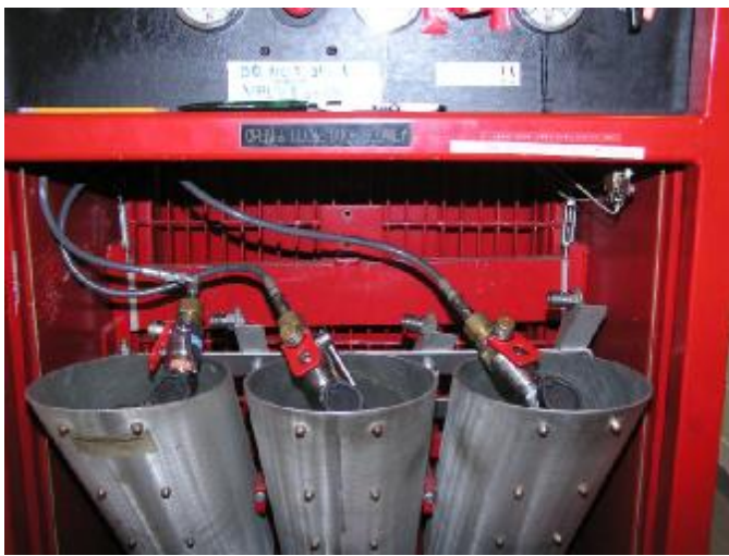
New method of positioning hose with right angle elbow pointed to the left..
